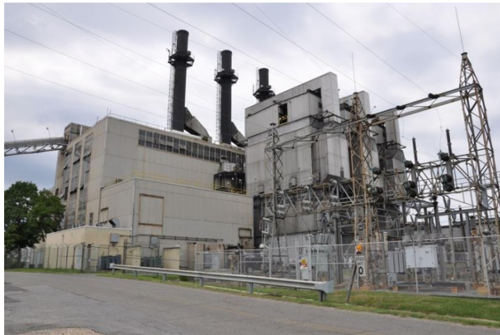
Goddard Power Plant, the last coal-fired power facility operated by the Navy, is being replaced in a $62 million military construction project on NSF Indian Head, MD. (U.S. Navy photo)
