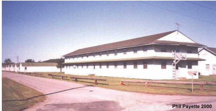
Barracks at Camp Pendleton
